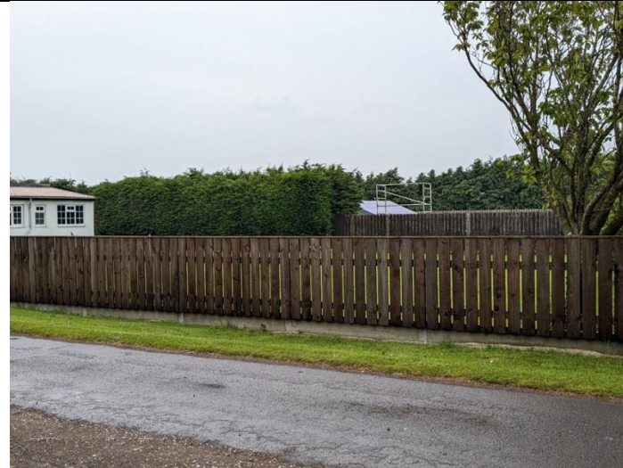
Left: South facing façade of the property.
